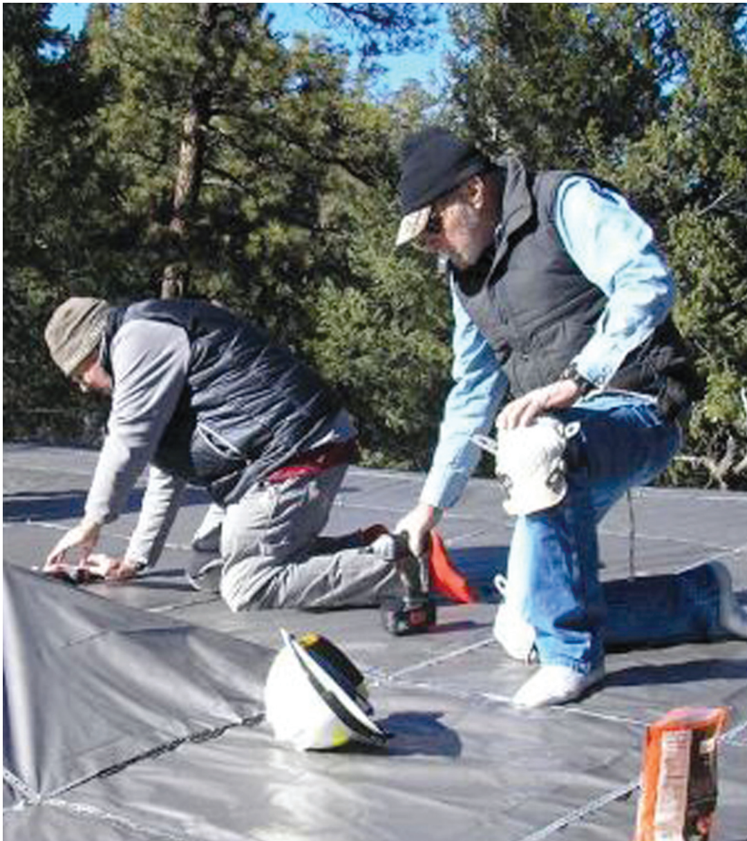
Figure 5. Mike and Lee Borduin installing heavy-duty tarp on unit house roof. Photo by Bill Cella.
